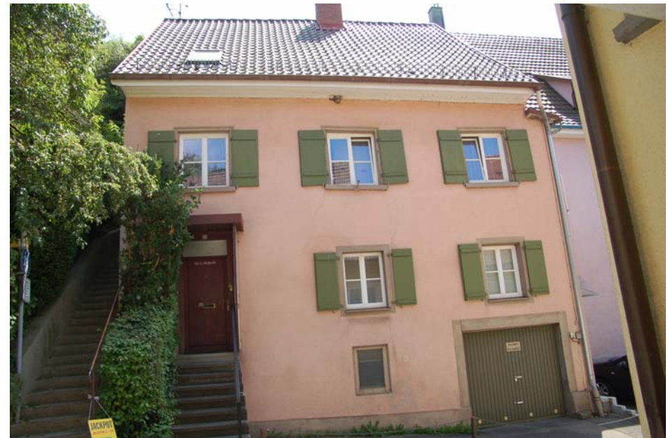
Frontalansicht (Foto: Ref. 26)
